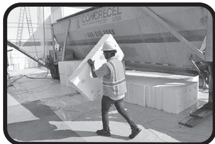
Construction improvements in progress
